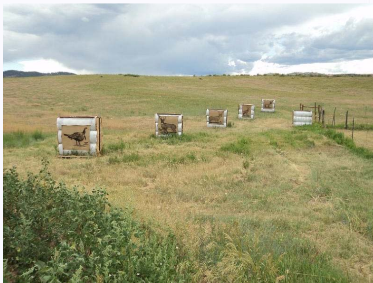
Work in progress on the new Archery Range.
